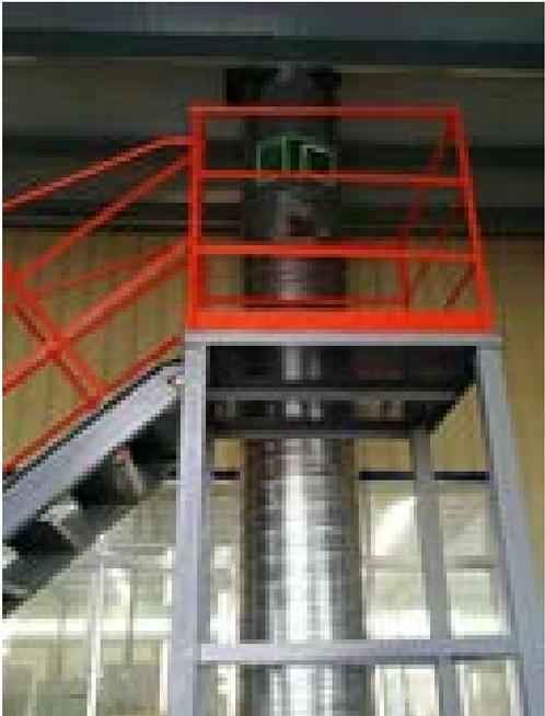
A photograph showing a UV light oxygen exhaust duct with a permanent monitoring platform and a pollution discharge port mark. The platform is made of red metal railings, and the duct is a large vertical stainless steel cylinder. The background shows an industrial setting with other equipment and a window. |
